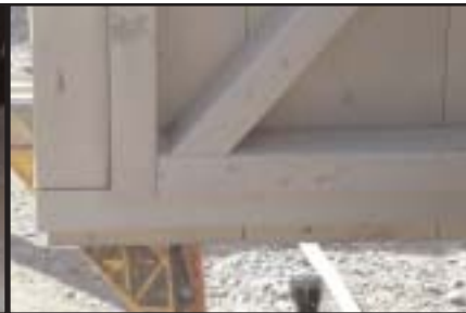
Fasten door stop to under side of door
