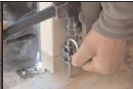
With barrel bolt locked in up position, space bolt and fasten on back of door one-finger width above floor
