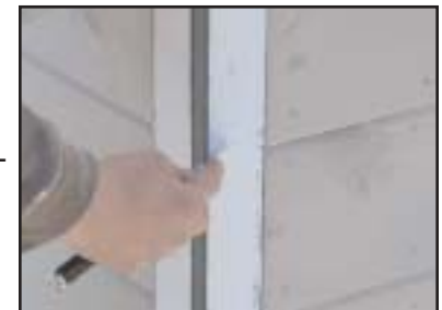
Putty holes & paint trim
