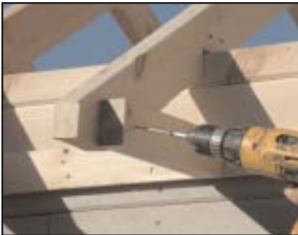
Attach roof rafters to braces
