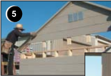
Fasten 2x4 on gable ends across sides
