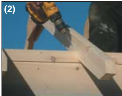
Fasten each rafter down (1) from the top and (2) from the side
