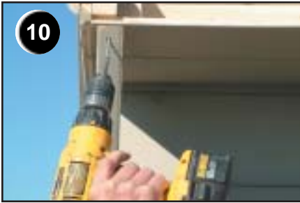
Fasten each overhang bracke into overhang board and front panel
