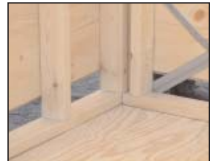
Screw the end panels to the floor.
