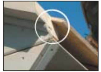
Roofing extends 1 1/2" over edge
