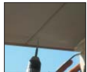
Make overhang board flush with bottom of rafter
