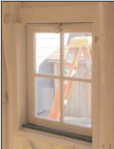
Fasten guides together with 1 1/2" finish nails
