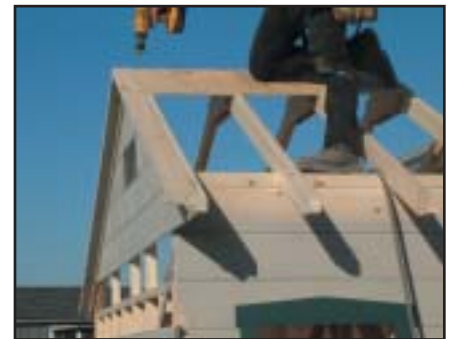
Apply plywood across peak of roof by screwing them into rafters
