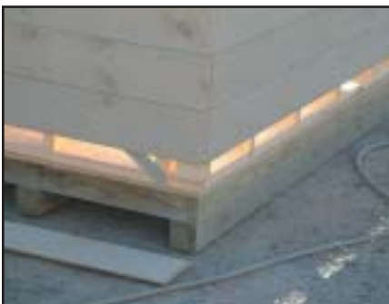
Apply lower siding boards around bottom of sheds
