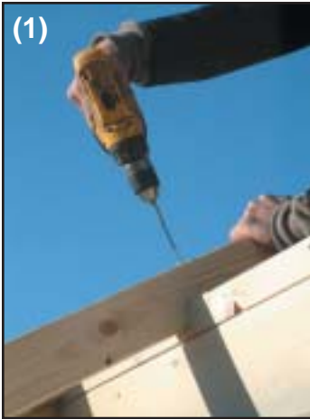
Fasten each rafter down (1) from the top and (2) from the side
