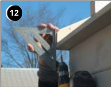
Square up overhang board for rear of shed & install
