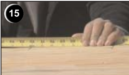
In center of roof at peak, mark cupola hole placement
