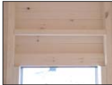
Install window guides against 2x4 provided
