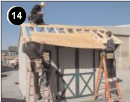
Install plywood roofing
