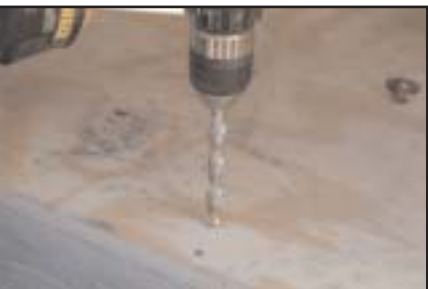
Where hammering the barrel bolt has dimpled the floor, drill a 7/16" hole, then hammer in the tee nut.
