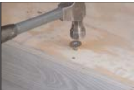
Where hammering the barrel bolt has dimpled the floor, drill a 7/16" hole, then hammer in the tee nut.
