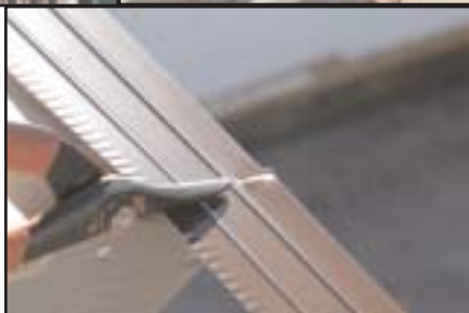
Cut & bend roof edging
