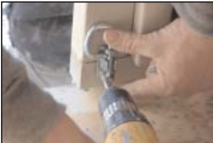
With barrel bolt locked in up position, space bolt and fasten on back of door one-finger width above floor
