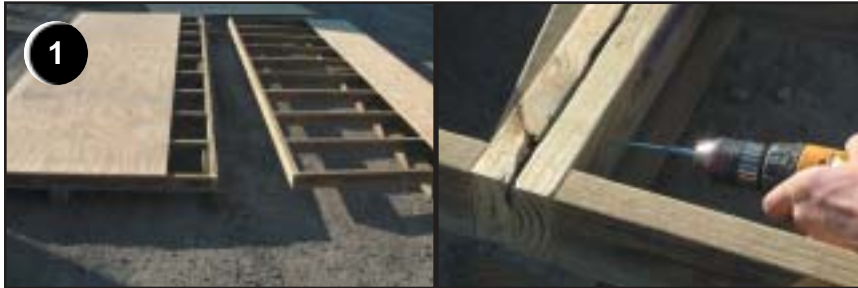
Join floor sections; screw sections together using two 3" screws on each side
