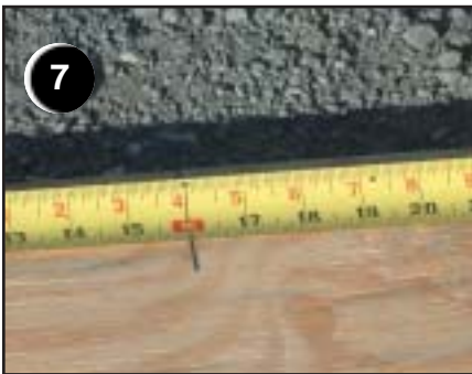
Mark plywood roofing 16" on center before installing
