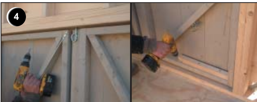
Unscrew doors at the top and bottom
