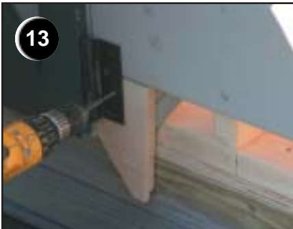
Unscrew bottom door hinges & remove spacers; insert bottom siding boards (shown marked)
