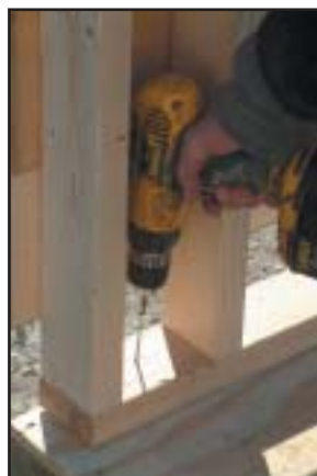
Attach front panel to floor
