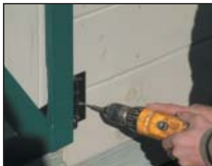
Re-attach door hinges
