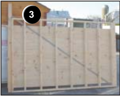
End panel. Note the 2x4s attached at either end.
