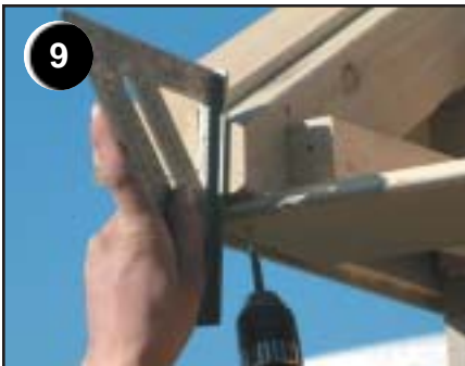
Square up overhang board & fasten in place
