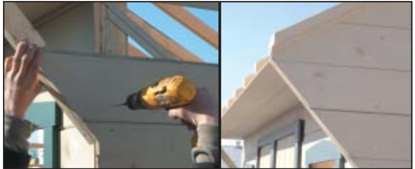
Apply & fasten side boards
