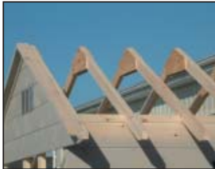
Rafters shown installed
