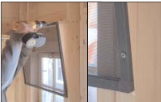
Install screens at top of window guides
