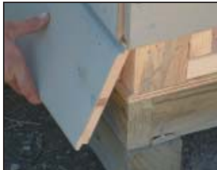
Unscrew bottom door hinges & remove spacers; insert bottom siding boards (shown marked)
