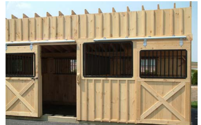
Sliding Stall Doors To Inside Isle
