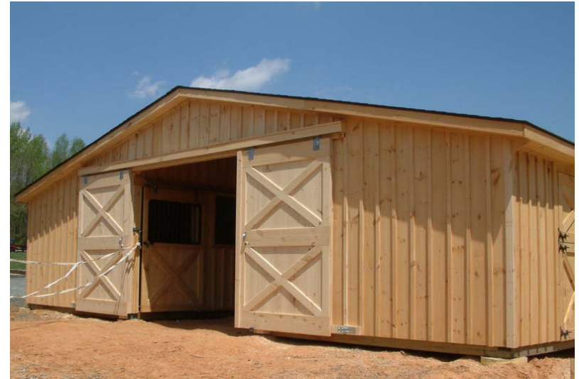
Roof Joined and Large Sliding Doors Added
