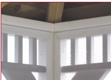
Figure 5i Two screen panels spaced in place before corner strip is installed
