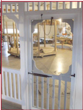
Figure 5e Interior of screen door with hardware installed
