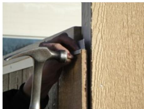
Note: Also you need to nail the siding down at the corners and along the bottom where it overlaps the floor.
