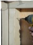
Applying screws to the adjoining wall studs.
