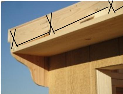
Place the soffit up against the re-tension strip and the ends of the roof rafters and screw in place by placing screws into the re-tension strip as well as the ends of the rafters.
