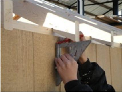
Place a square against the siding and the tip of the roof rafters (as shown) and scribe a line across the front and back wall.
