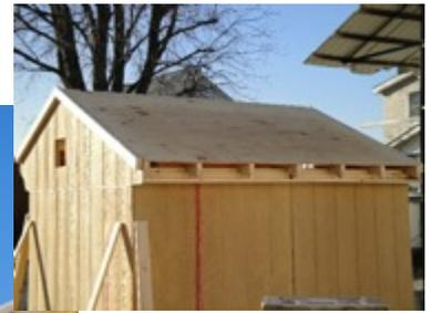
Apply the plywood roof panels - lay the panels on the roof and square the up to the ends of the rafters as shown, Then screw them in place using the 2" screws.
