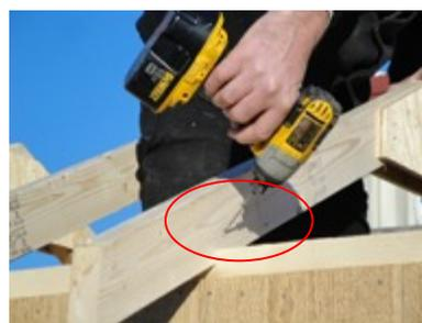
Space out the pre-assembled roof rafters on the headers as marked. Note: the notches in the rafters will hold them in place until you fasten them.
