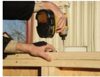
Lay the shorter 2 x 4 top wall plate across the top of the back wall. Center it on the wall so that there is a gap at the ends (as shown) and screw in place.
