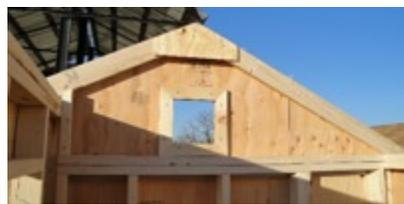
Set the pre-assembled gable ends (note: end vents will be installed) on top of the side wall and butt fit the panel against the front wall on the Quaker and screw in place using the 2½” screws (to the front wall on the Quaker as shown and along the top of the wall section).
