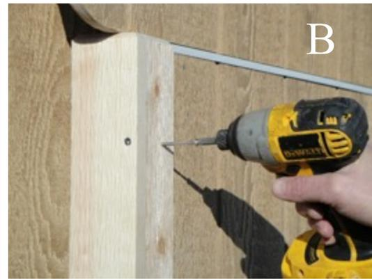
First screw the two corner strips together at 90 degrees to each other as shown in photo "A" then fasten to the shed as shown in photo "B"
