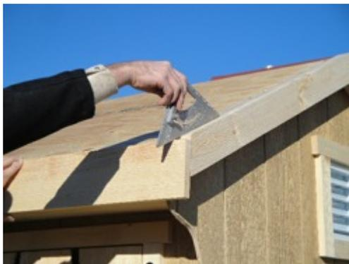
Square up the fascia plate with the roof sheathing and screw in place on both the front and back of the shed. Place the screws into the ends of the rafters. Now your shed will look like this.
