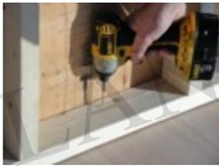
Applying screws to the sill plate and into the floor.
