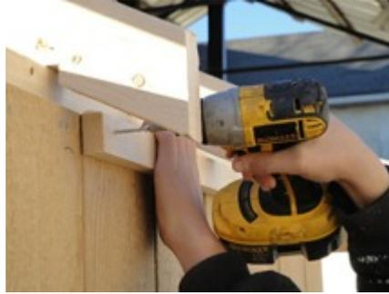
Place a 1 x 2 soffit re-tension strip above the line and screw in place (as shown).
