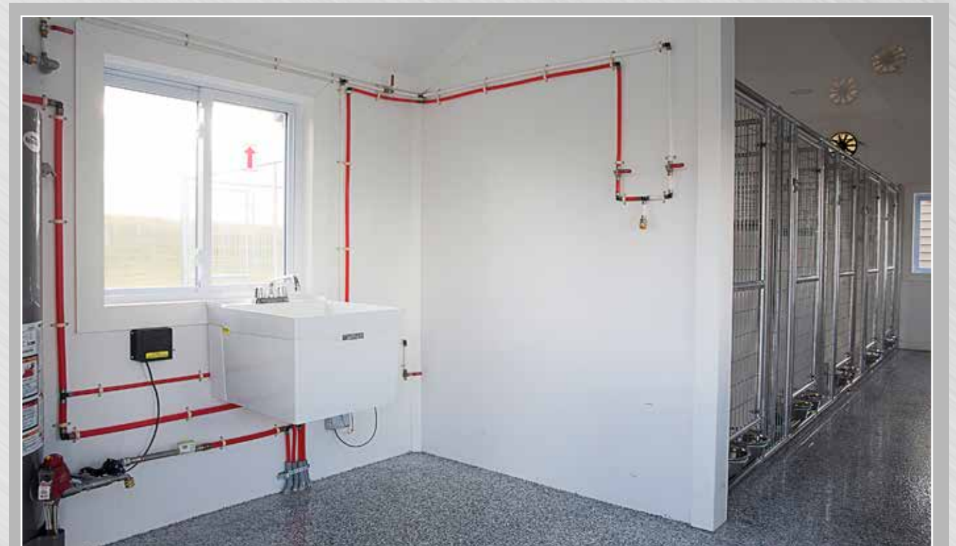
Interior View Of 10x28 showing optional floor heating, utility tub, hose port, welded wire panels with feeder bowls in gates
