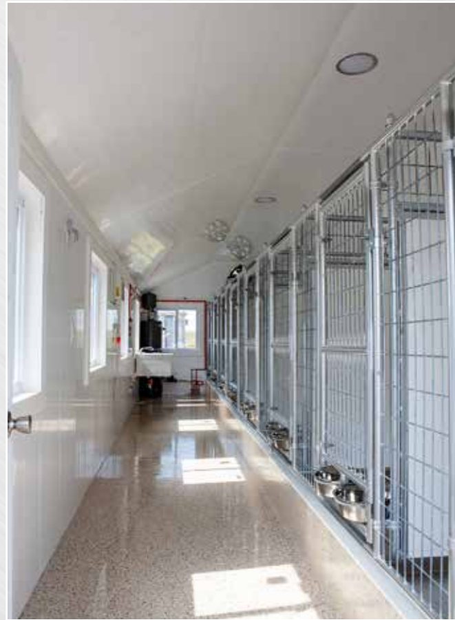
Interior View Of 14X32 Showing Optional Raised Floor, Feeder Bowls, 4'High Solid Divider, Welded Wire Panels, New! Stainless Steel Wash Down Trays In Dog Boxes
