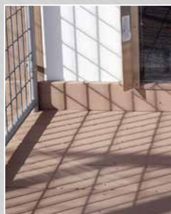
PVC Decking on Runs
