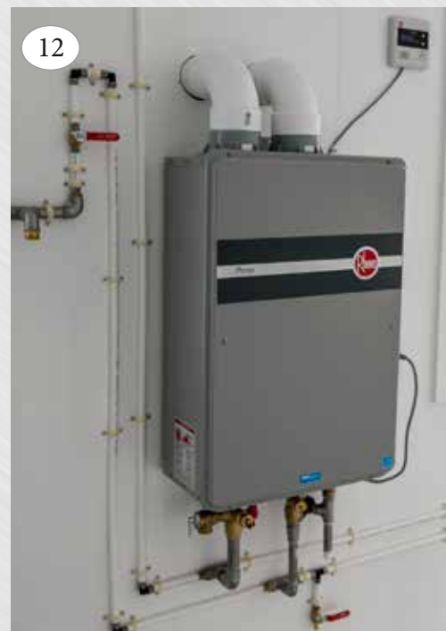
12 On Demand Water Heater Uses LP and Electric
