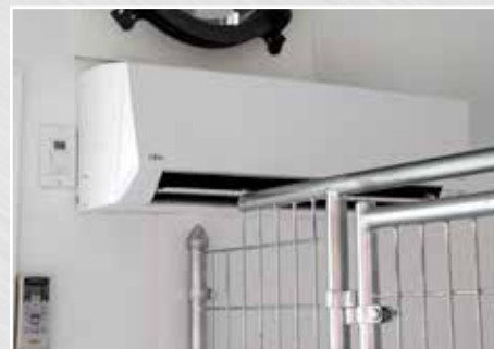
Interior View of Mini Split Heater/AC Unit
